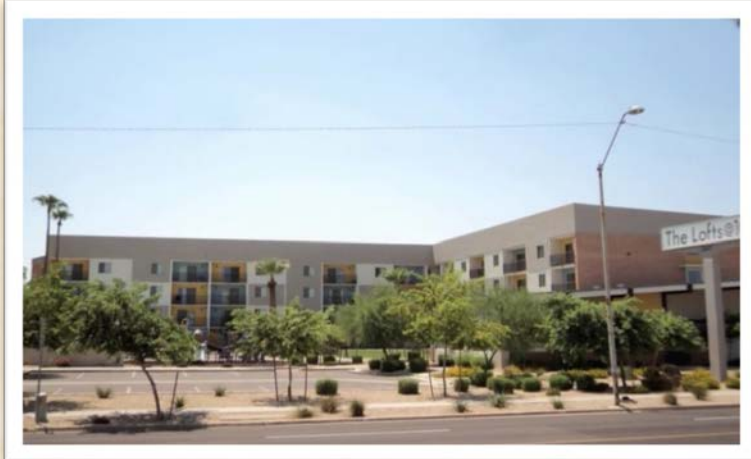
UMOM – Family Shelter City Council Dist. 8 33 rd and Van Buren Streets
